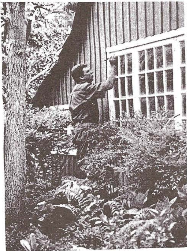
BY THE NUMBERS — Bill Abel hand-numbered every board of Walt Disney's train barn before dismantling it. He expects the reconstruction and installation of the building near Travel Town in Griffith Park to be complete by August.
